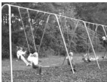
If there are more than two swings in a bay, remove the middle swing(s).
